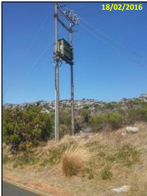
Figure 8: H-Pole at the Brooklands Waterworks where the juvenile baboon was electrocuted.
